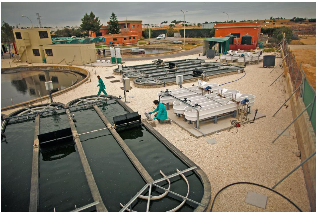
The goal of All-gas is to produce 3,000 kilograms of dry algae annually with an oil content of 20 percent. That would be enough biodiesel to fill the tanks of about 200 cars. Bio-methane production from anaerobic digestion and sludge residue is expected to provide an equivalent amount of bio-methane for another 200 cars. The plant would eventually cover 10 hectares of land if it moves beyond the five-year pilot.
